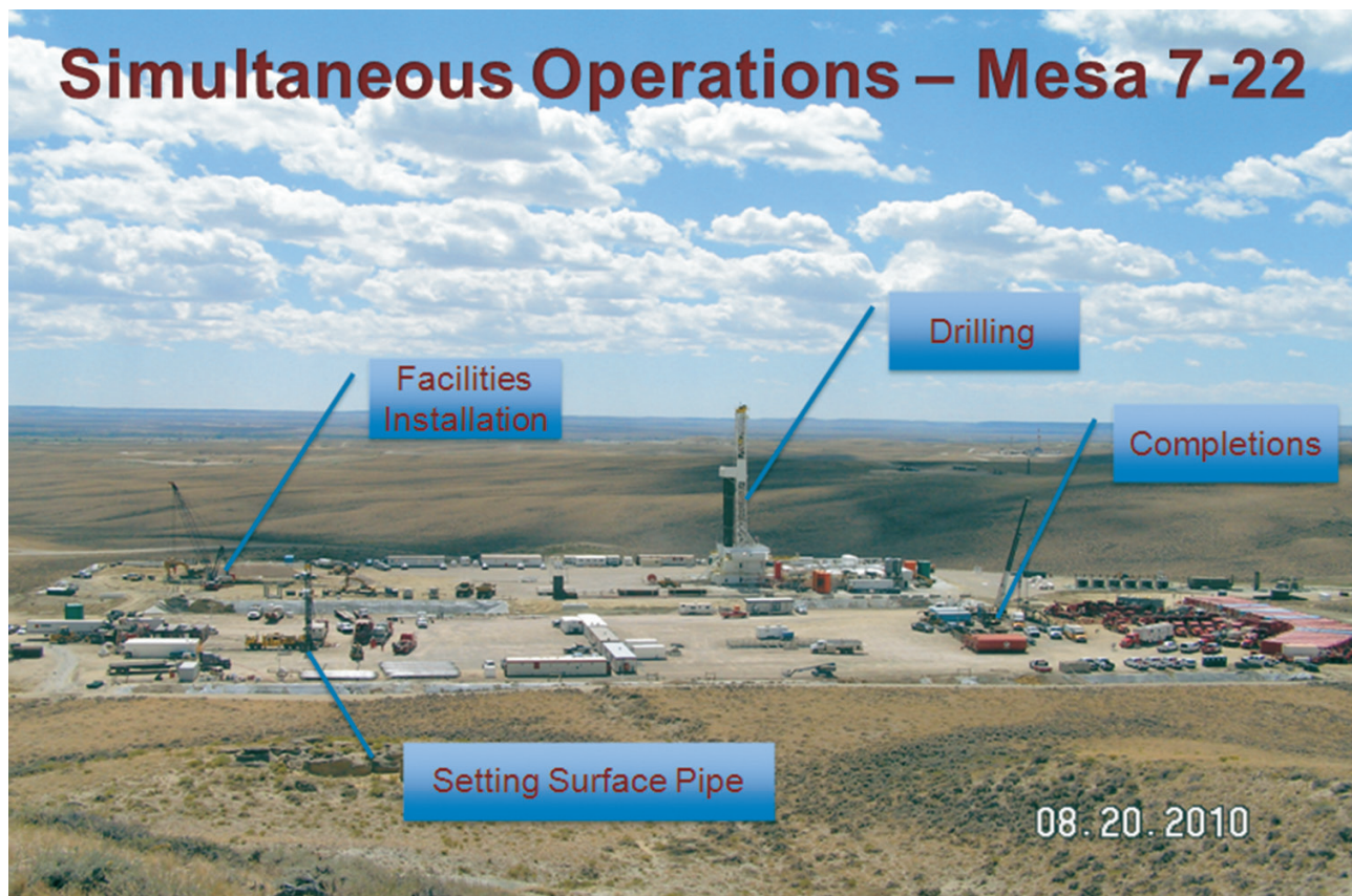
Figure 3. Simultaneous operations being conducted in Pinedale field with drilling, fracking, setting of surface pipe, and facilities installation all occurring concurrently.
